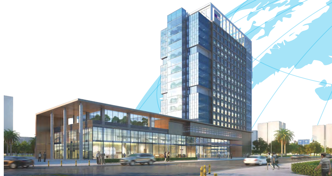
库马克智能驱动与自动化研发总部基地 Cumark Intelligent Drive and Automation R&D Headquarters Base
